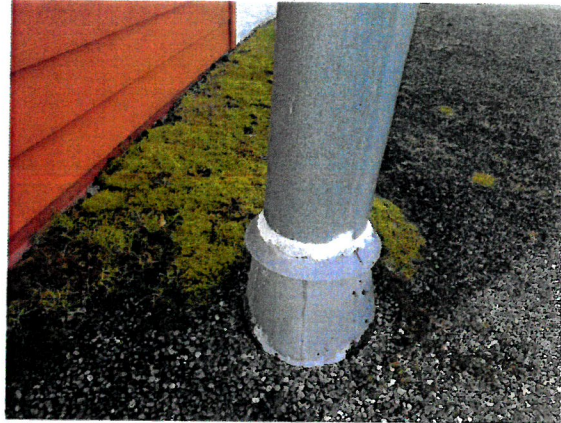
Photo 20: Caulking – Roof on Vent (ND)
