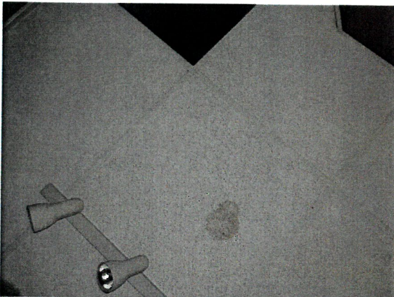
Photo 15: Ceiling Tile – Throughout Main Floor (ND)
