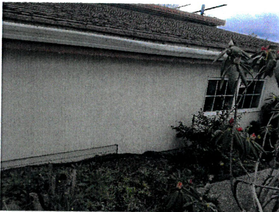
Photo 27: Stucco – Exterior Side (ND)
