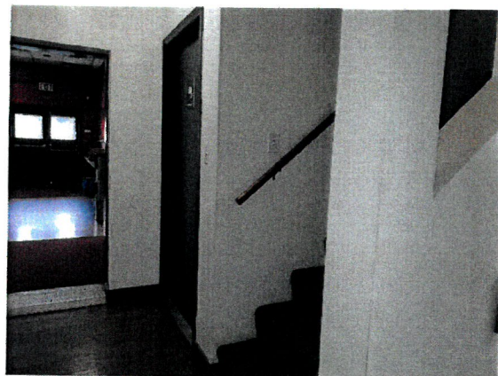
Photo 6: Drywall Compound – Stairs To 2 nd (ND)
