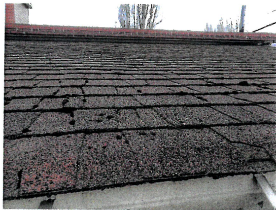
Photo 24: Composite Shingle – Gym Addition (ND)
