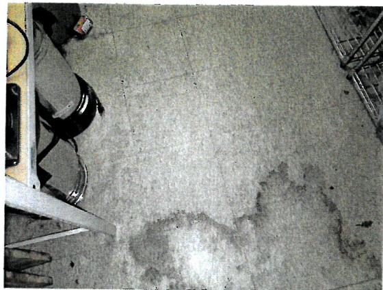
Photo 12: Vinyl Floor Tile – Kitchen Storage (ND)
