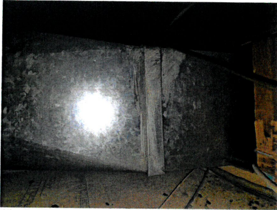
Photo 19: Mastic – HVAC (ND)
