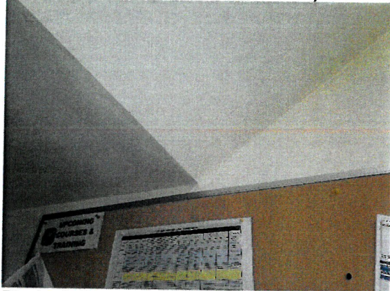
Photo 1: Drywall Compound – Main Floor Stairs to Truck Bay (ND – none detected)
