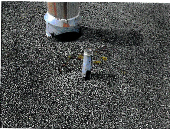
Photo 21: Tar – Roof on Vent (ND)
