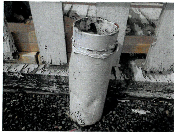
Photo 22: Caulking – Roof on Vent (ND)
