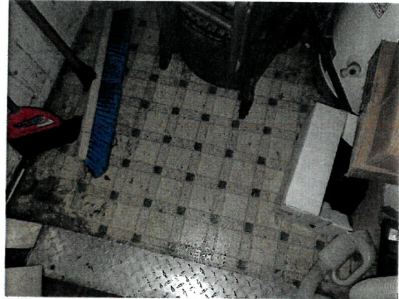
Photo 14: Sheet Vinyl Flooring – Cleaning Closet (ND)
