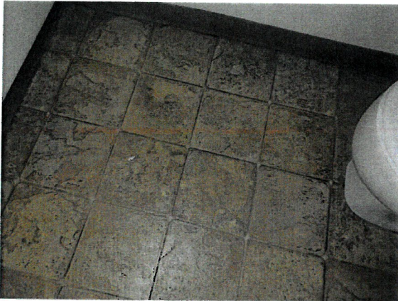
Photo 13: Sheet Vinyl Flooring – Washroom (ND)
