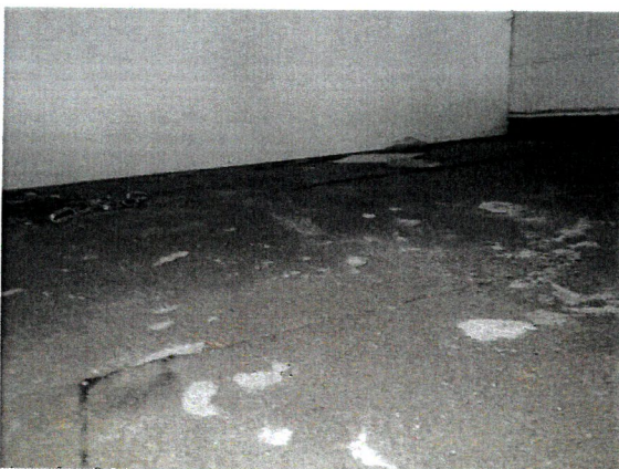
Photo 23: Torchon Membrane Roofing – Gym Awning (ND)
